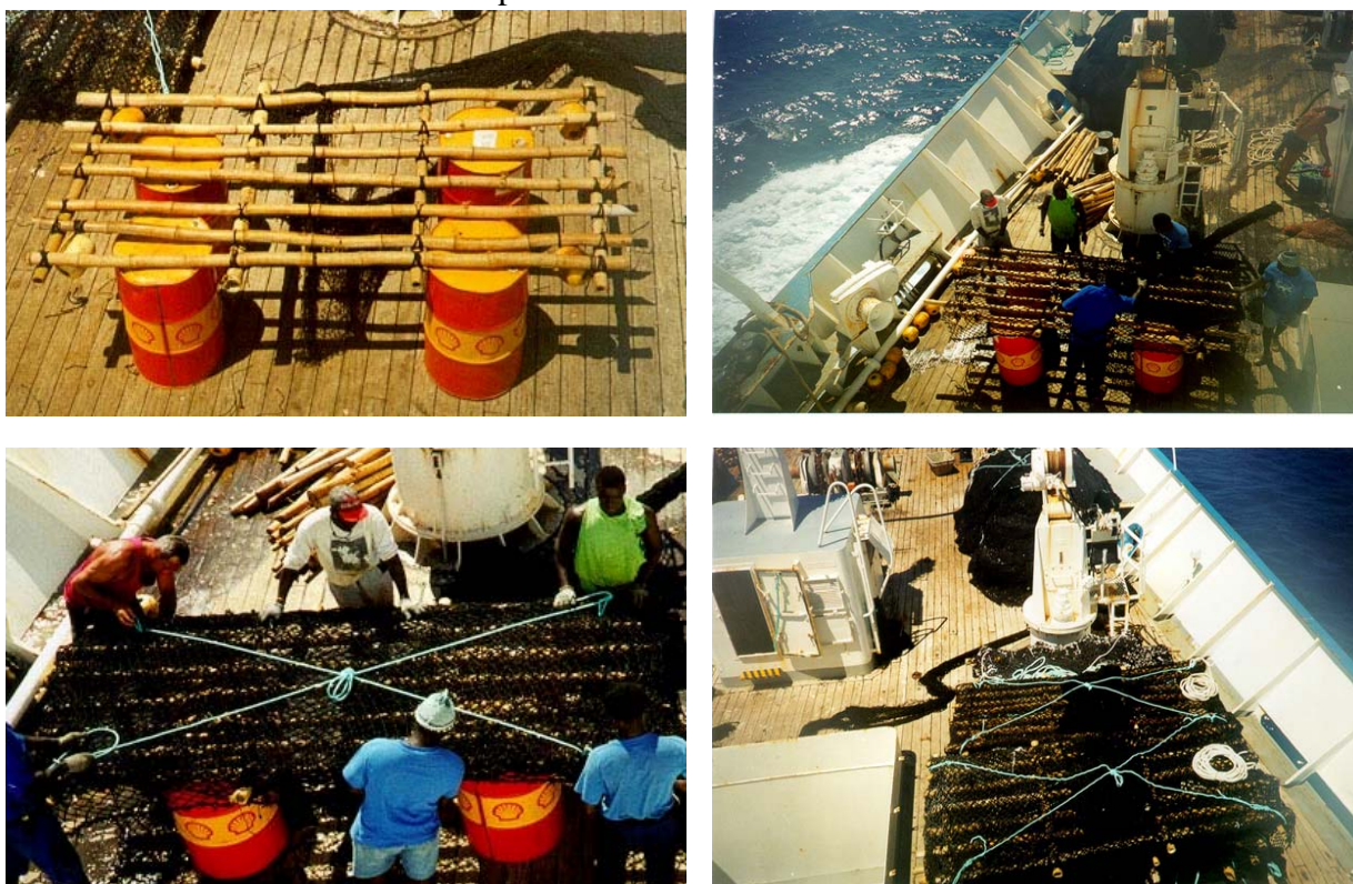
Fig. 4. Building a FAD (© AZTI/isancristobal).
