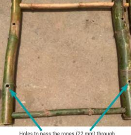
Holes to pass the ropes (22 mm) through to connect the 2 bamboo frames.
