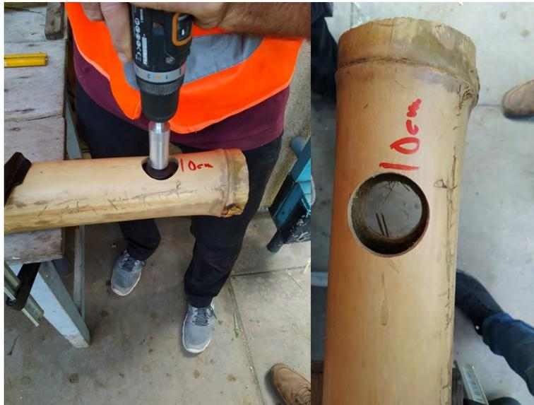
4. Drill a whole of about 20mm diameter through the bamboo cane on both sides (for the rope)
